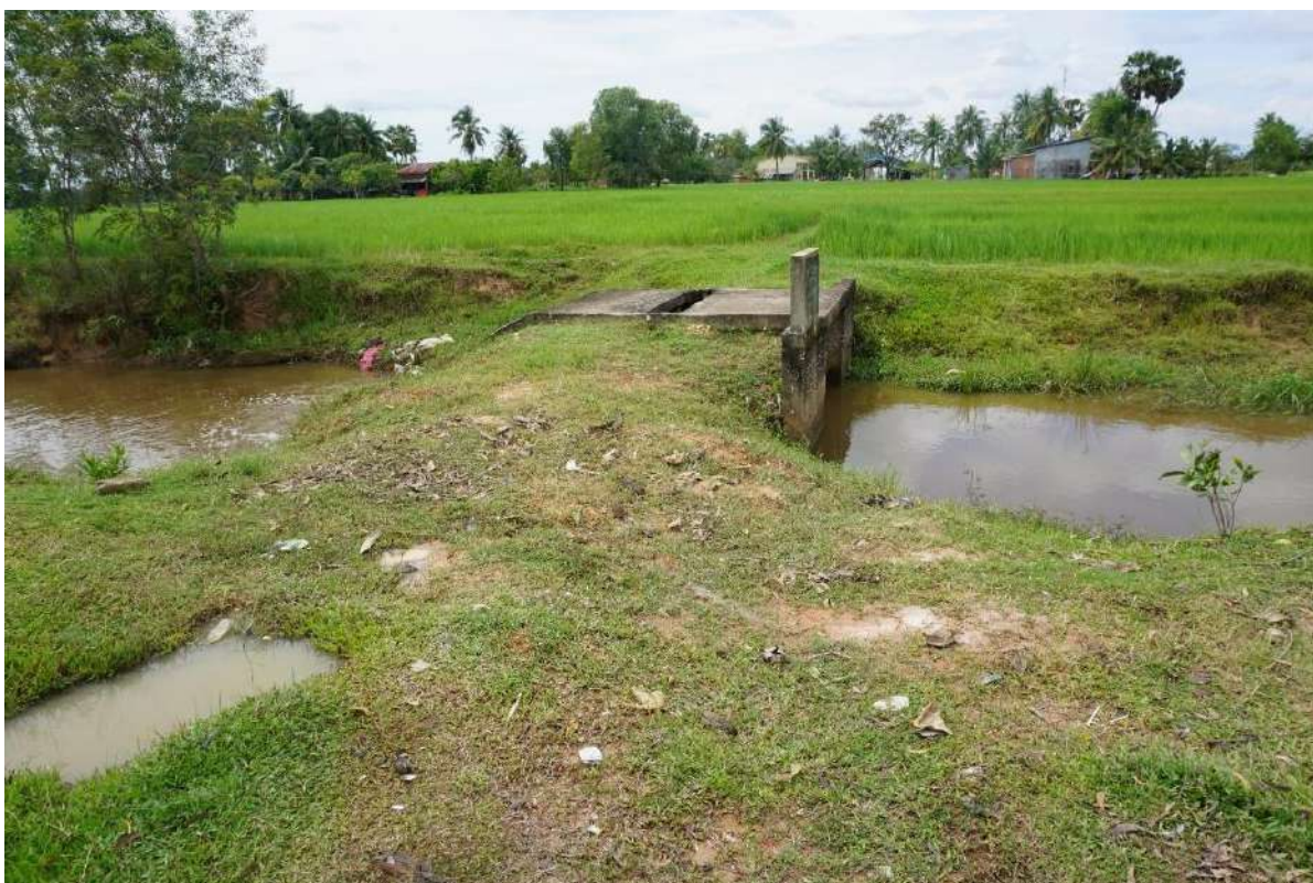
Figure 17 “Eroded embankments around water gate 1”
