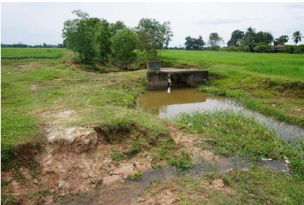
Figure 15 “Erosion embankments water gate 1”
