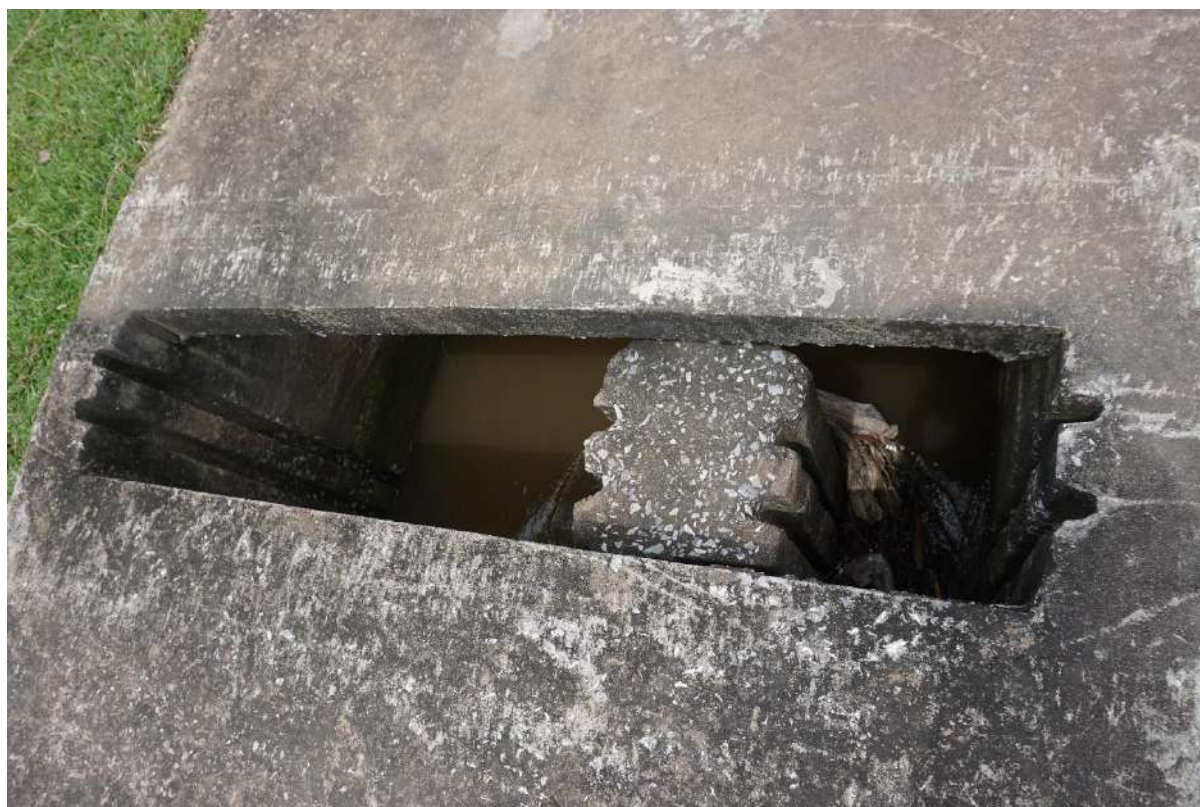
Figure 4 “Missing spindle in gate 1”
