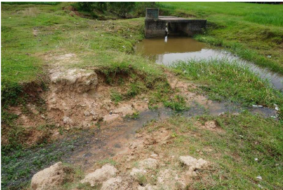
Figure 14 “Erosion upstream water gate 1”
