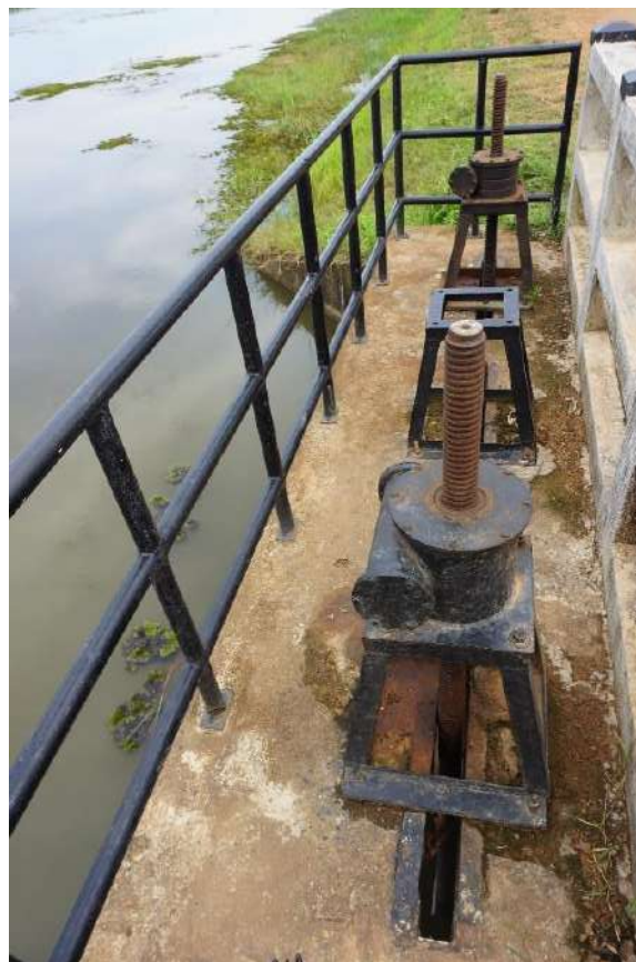
Figure 7 “Double sluice gate east O Thmar Reservoir”
