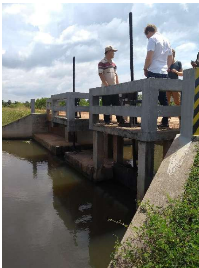
Figure 7 “Photo 3 – typical sluice gate as used elsewhere in Angkaol – use same standard design for the vertical lifting gates in this sub-project.”
