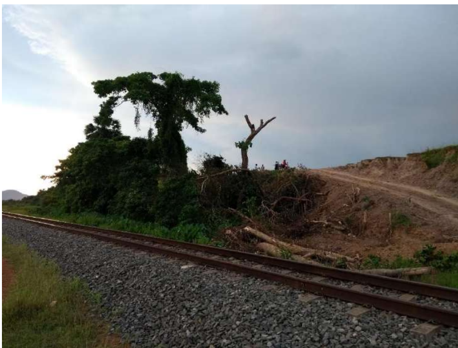
Figure 6 “Downstream face showing access road ramp up to crest, dense vegetation and proximity of railway line.”
