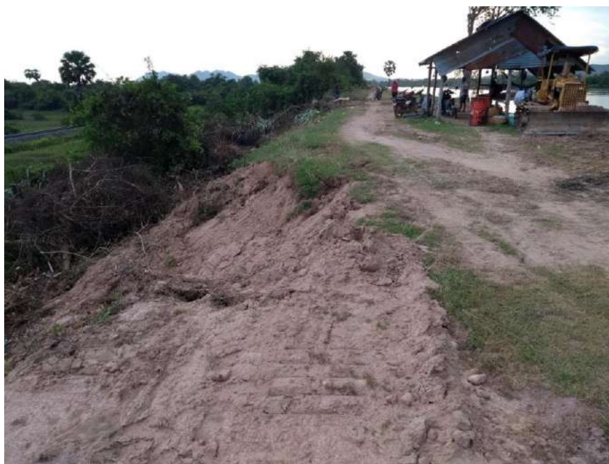
Figure 3 “View along the crest of the dam showing eroded embankment face and vegetation on the downside of the dam”
