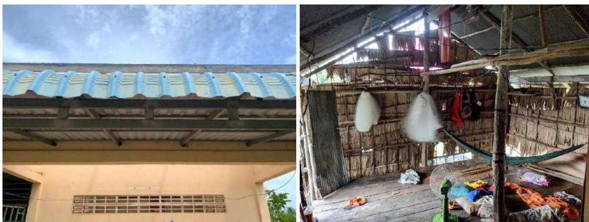
Figure 10 “Example of higher quality corrugated sheeting construction. Use of screws with washers evident. Higher quality corrugated steel noted as composed of thicker material.”
