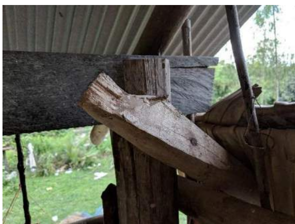
Figure 18 “Example of poor joint construction with inadequate materials and construction quality. Example of poor joint construction.”
