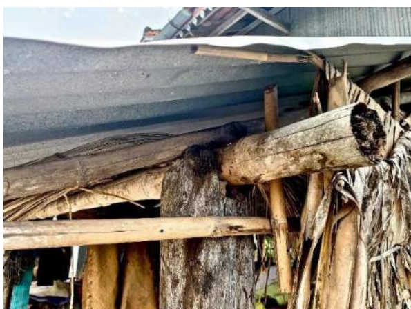
Figure 18 “Example of poor joint construction with inadequate materials and construction quality. Example of poor joint construction.”
