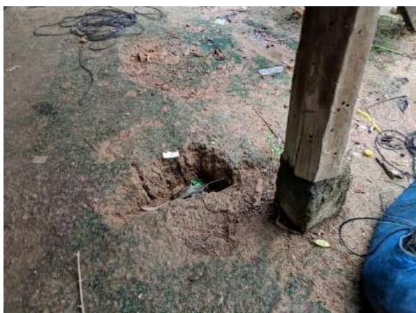
Figure 16 “Closeup of foundation failure identified in Figure 10. Foundation not secured into ground with evidence of previous failure.”
