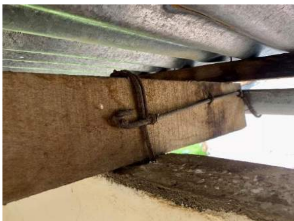
Figure 22 “Example of poor joint construction with inadequate materials and construction quality.”
