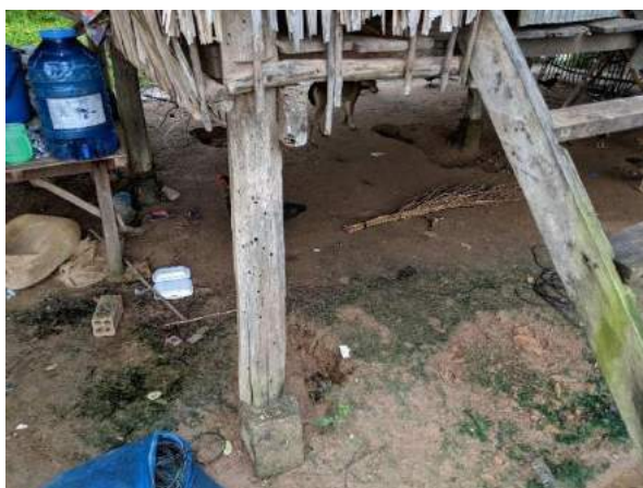
Figure 16 “Closeup of foundation failure identified in Figure 10. Foundation not secured into ground with evidence of previous failure.”
