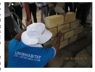
Mud concrete technology is both cost effective and environmentally friendly. Having been subjected to rigorous laboratory and field testing, it is proven to be of good strength with the ability to withstand extreme weather
